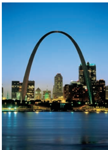
Glen Allison/Stone/Getty Images The design of the Gateway Arch in St. Louis is based on an inverted hyperbolic cosine curve (Exercise 73).
